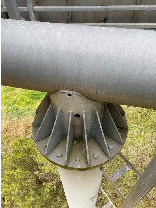
Photo 1 – Monopole to torsion beam flanged connection.
