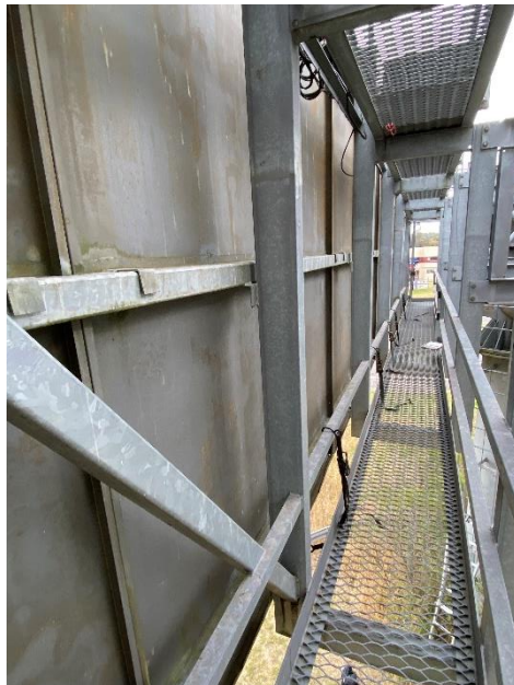
Photo 8 – General view of bottom gantry
