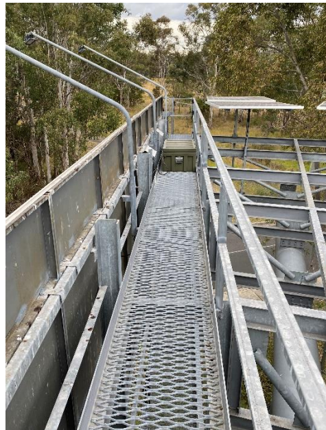
Photo 9 – General view of top gantry
