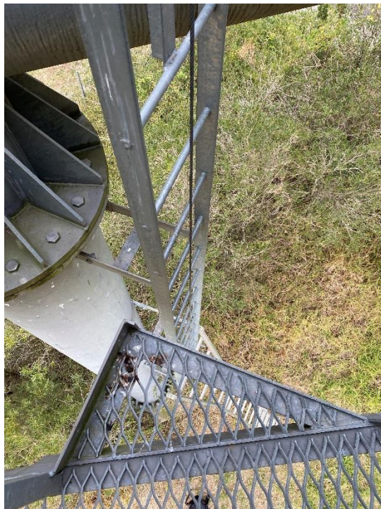
Photo 3 – Vertical access ladder equipped with `Ladsaf`.
