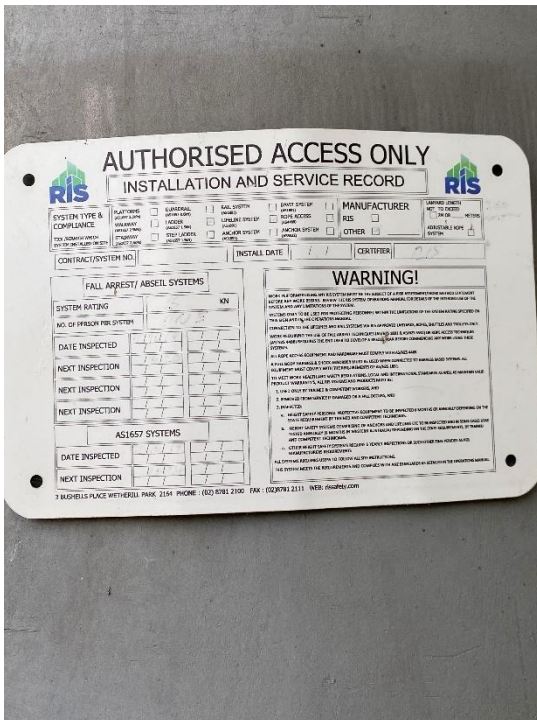
Photo 4 – ‘Ladsaf’ installation and service record affixed to the structure.
