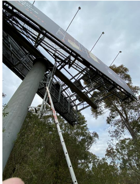
Photo 7 – General view from underside
