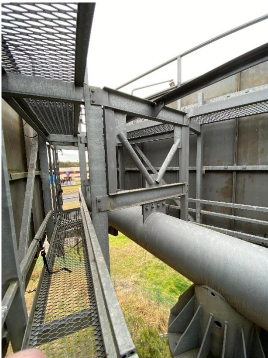
Photo 2 – Typical trussed frame connected to top of torsion beam.
